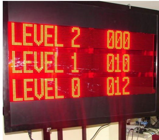
Figure 2.3.1.4: Parking Entrance Display
