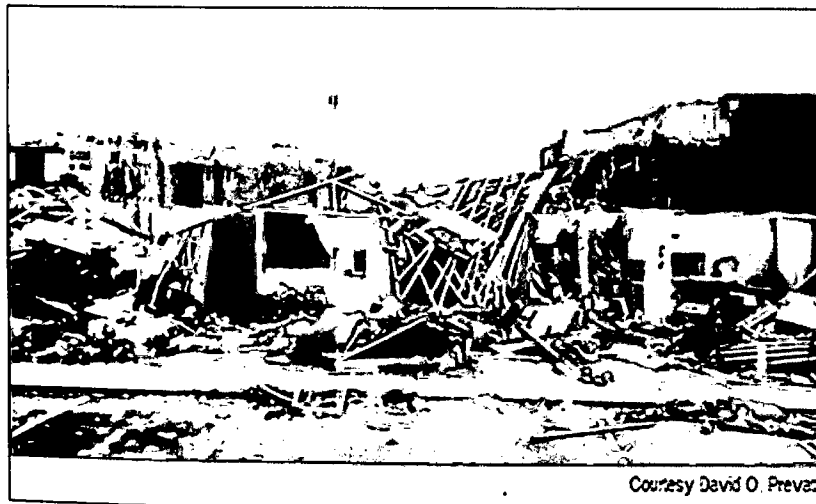
Figure 2.5: Damage for whole roof structure.
